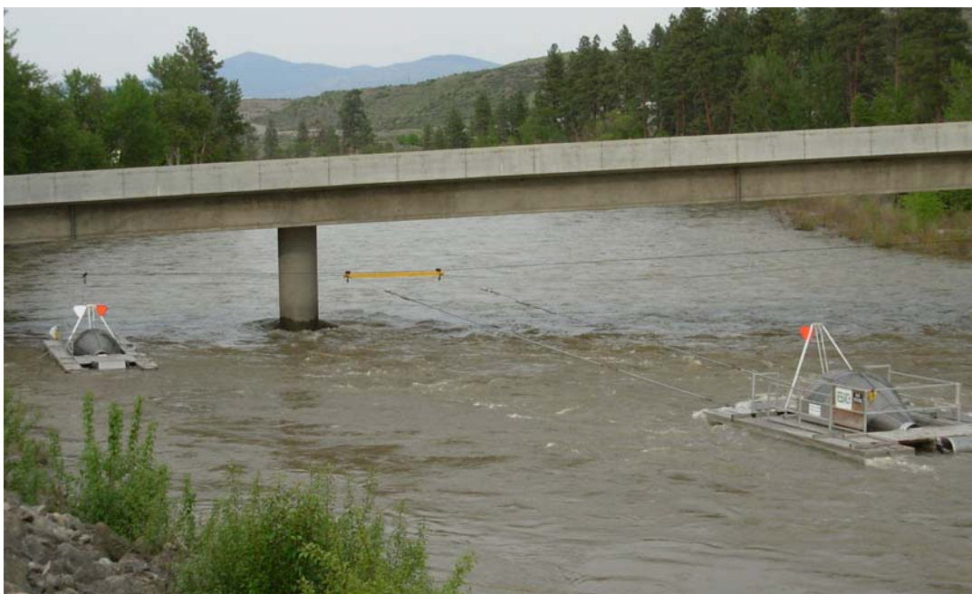
Figure 3. Photograph of the 8-foot rotary screw trap in the main channel (right) and the 5-foot rotary trap in the secondary channel (left) at 9,500 cfs.
